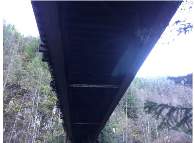
Main span superstructure
