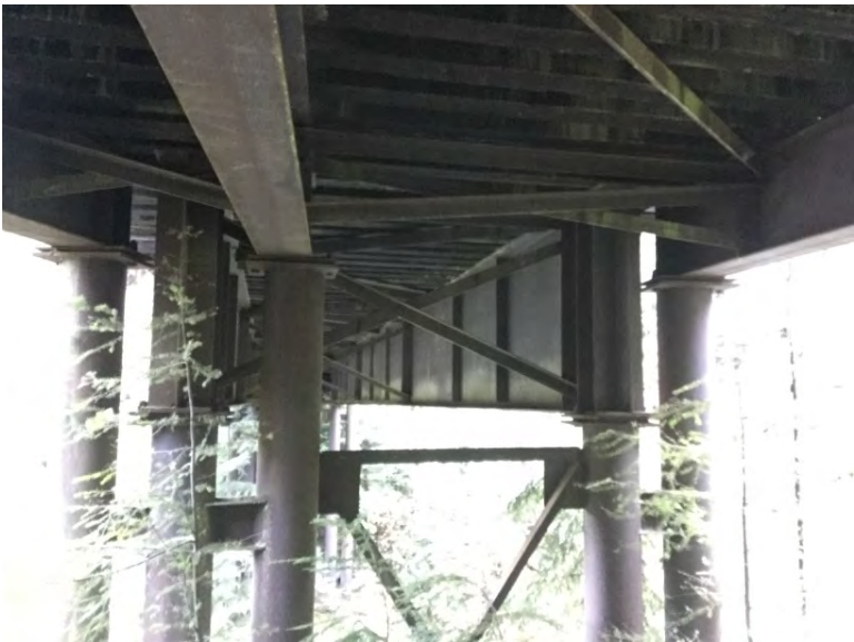
Bearings at left Pier
